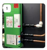
1. Ensure all plumbing isolation valves are fully open and the cold water storage tank is 100% full. Image depicts a typical wall-mounted SmartValve™ installation where the outlet pipework is rising to the outlet accessory in the bathroom.
