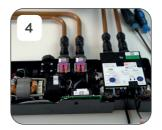
Remove the cover from the SmartValve™.
